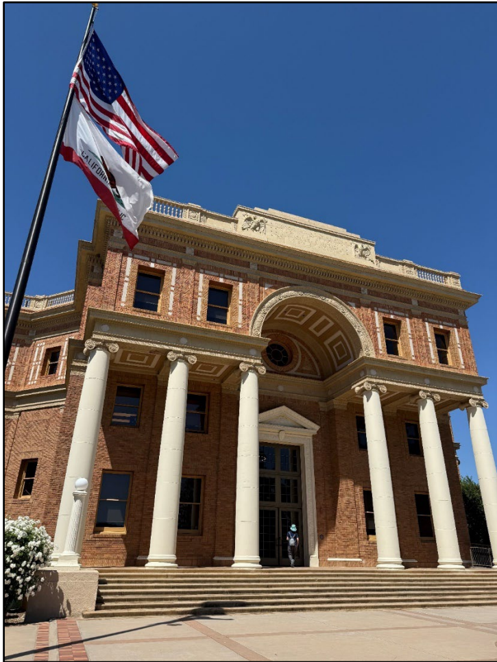
Figure 4.1-2. Photograph of Atascadero City Hall (June 20, 2025).
